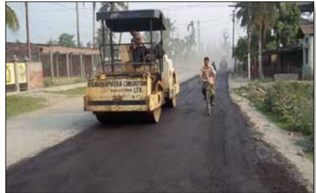
Compaction of Cold Mix
