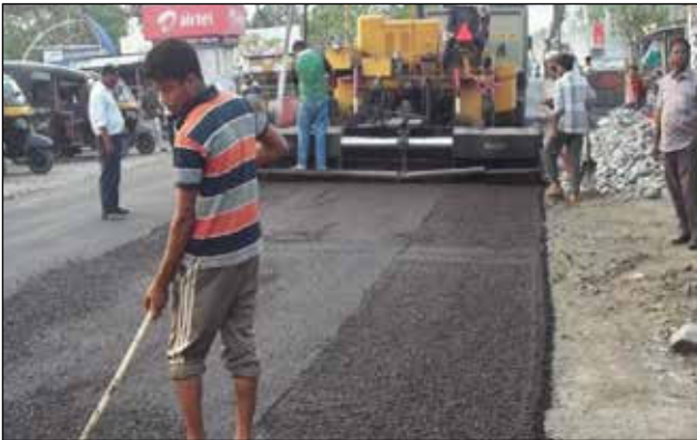
Laying of Cold Mix with Paver
