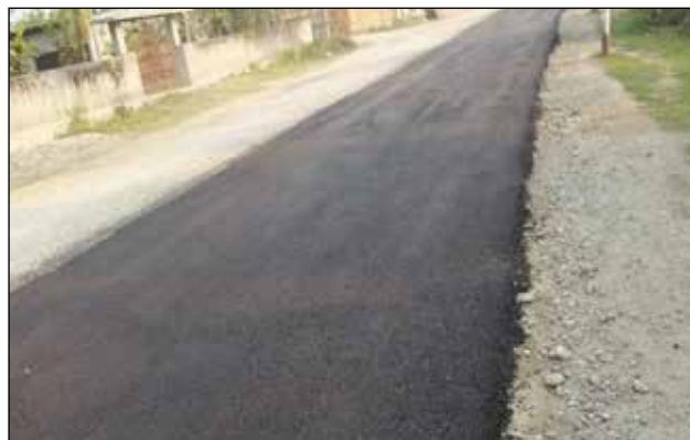
Cold Mix Road Finished Surface
